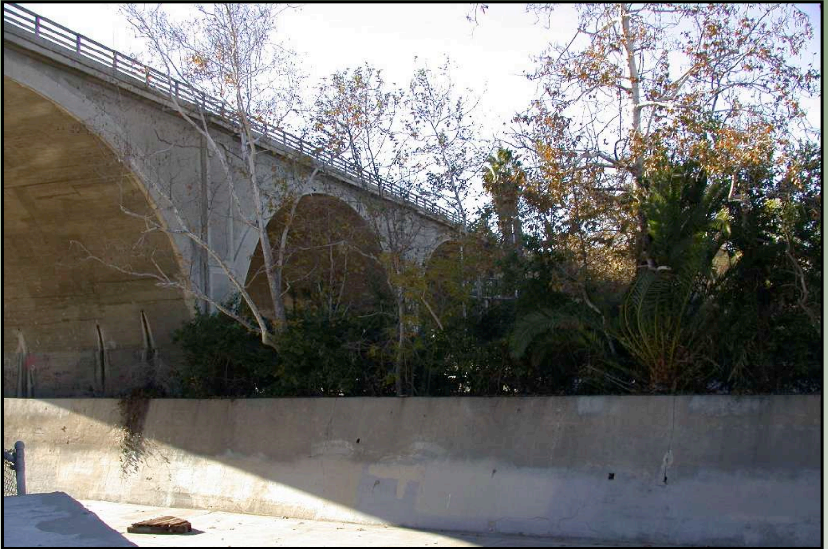
York Street Bridge in 2003
