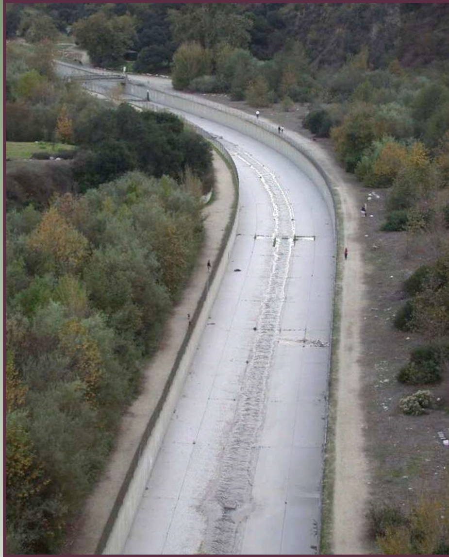
Box channel in Arroyo Seco.
