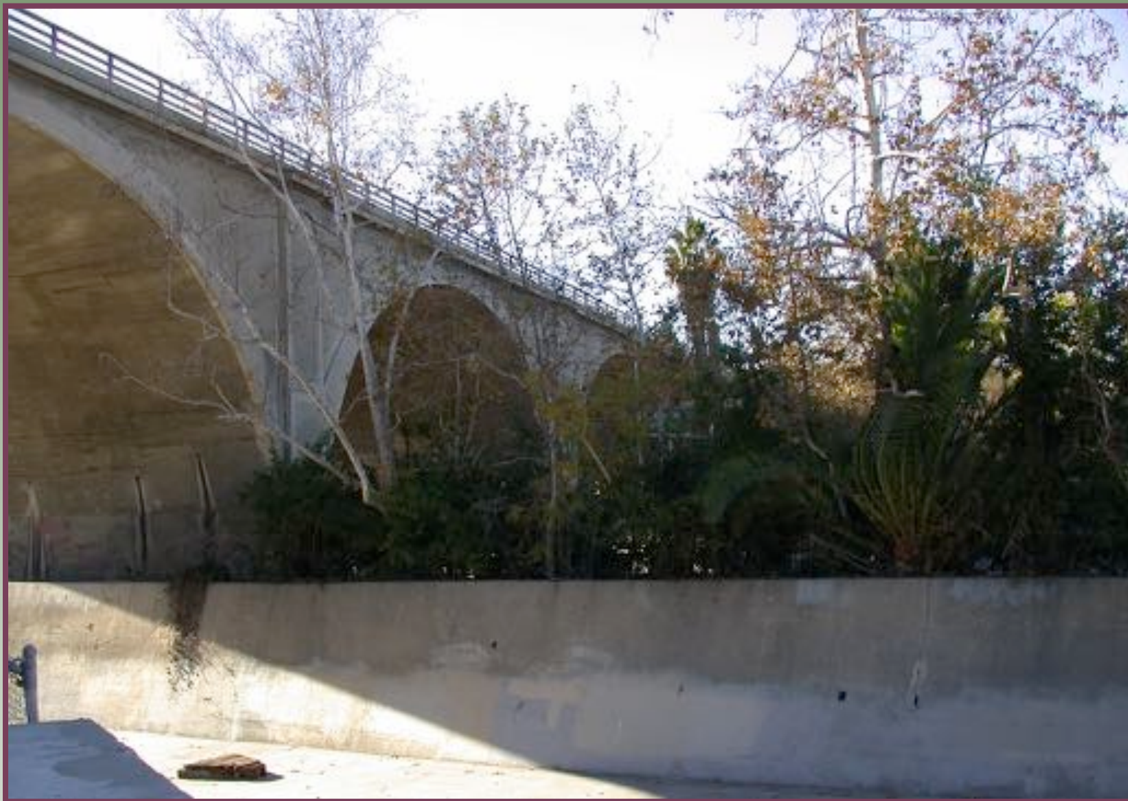
York Street Bridge in 2003
