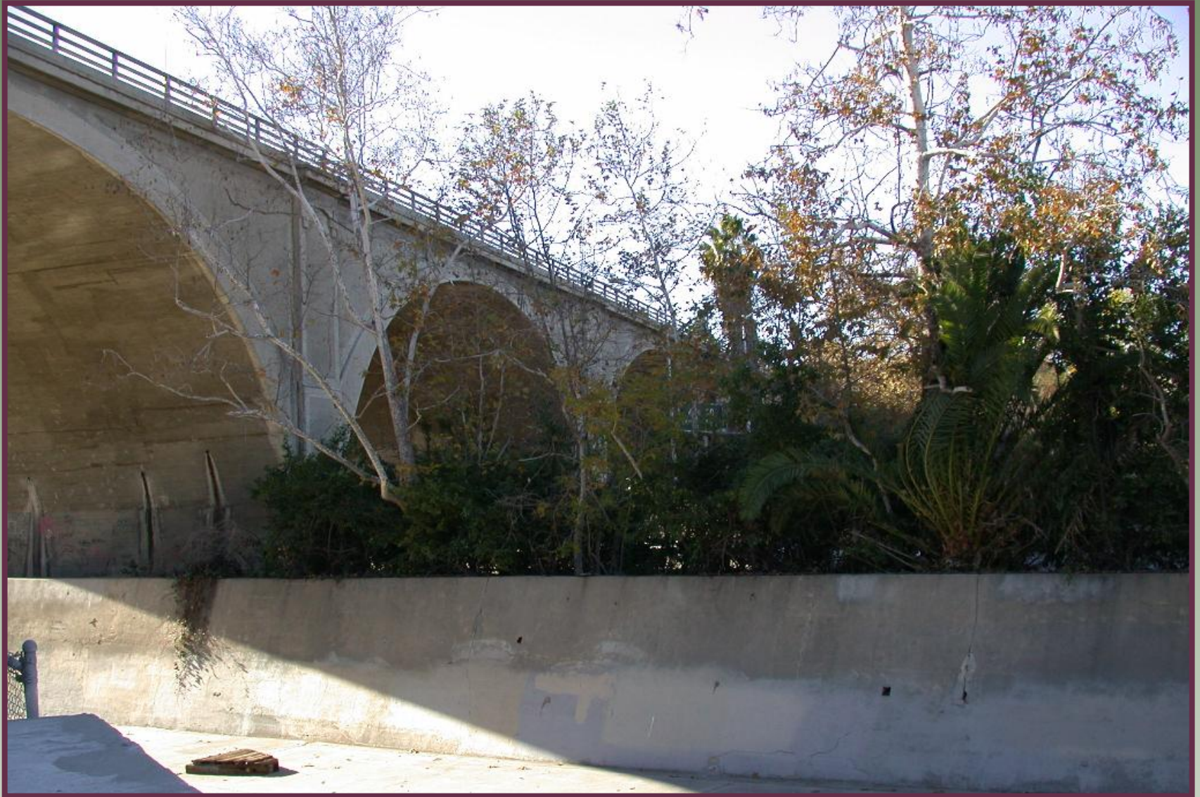
York Street Bridge in 2003
